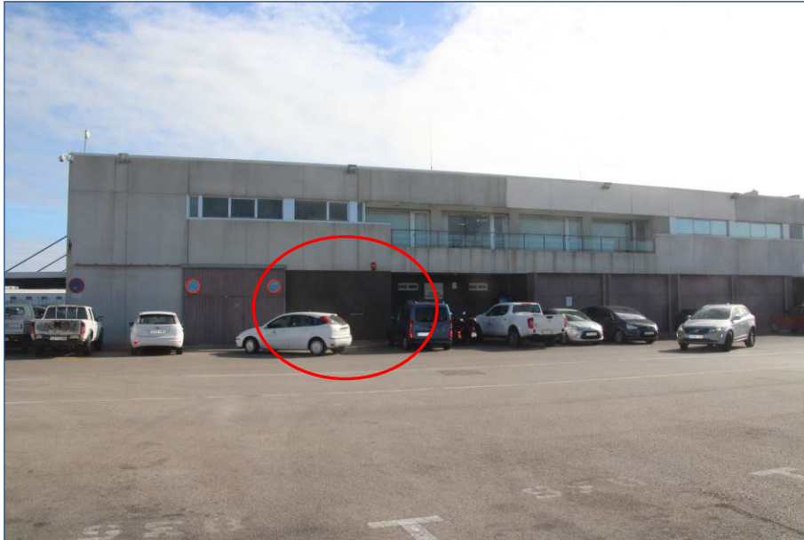
CBPA Safety and Environment Warehouse
