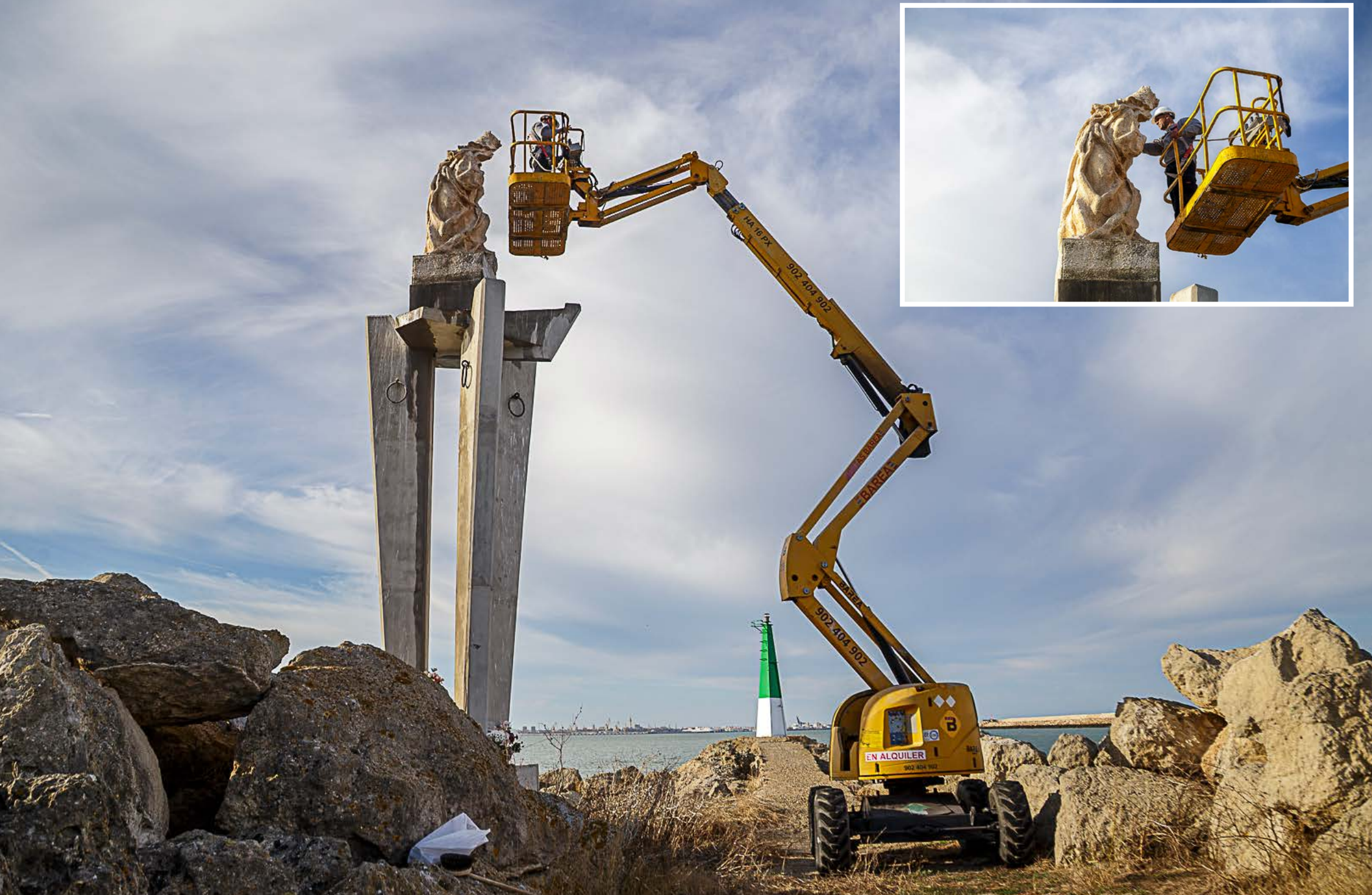
Conservation work on the statue of the Virgin of Carmen on the breakwater at El Puerto de Santa María. November 2025
