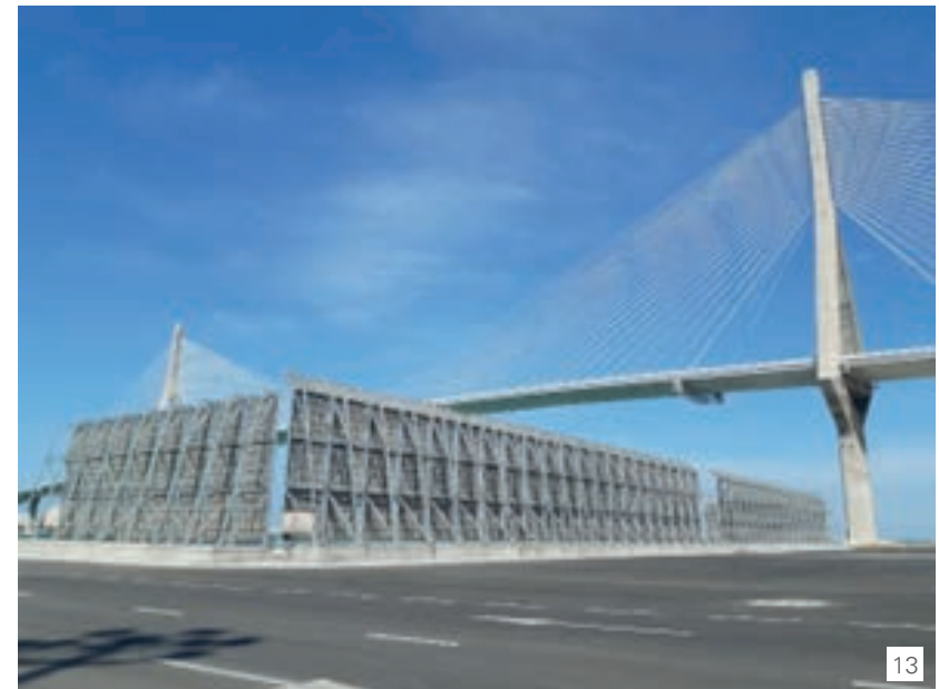
13. Since August 2020, the old screens have been replaced by a new configuration (left, old screens).
