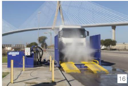
14. Implementation and maintenance of wheel washers. 15. Location of the wheel wash system. 16. Wheel washer in operation. 17. Proposed route.
